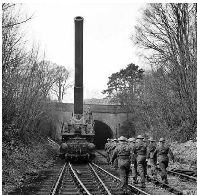
A drill session in progress as HMG Boche-Buster waits outside the south portal of Bourne Park tunnel in March 1941.
